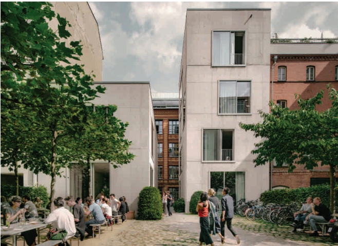
Referens genomsiktighet (Campus Joachimstraße, David Chipperfield).
