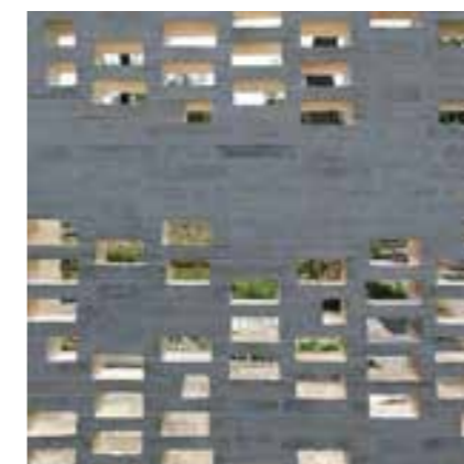
Referens perforerat tegel (Maggies Lanarkshire, Reich and Hall Architects)
