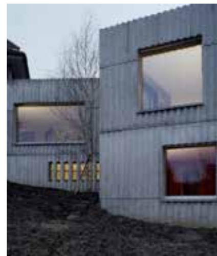
Referens betongsöcket (House extension and renovation, Christ + Gantenbein)
